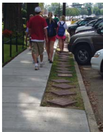
Some campus sidewalks are undersized for increasing pedestrian volumes.
